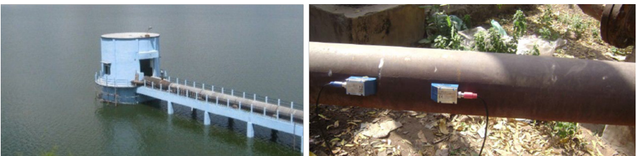
Figure 16: Intake well and portable flow meter
